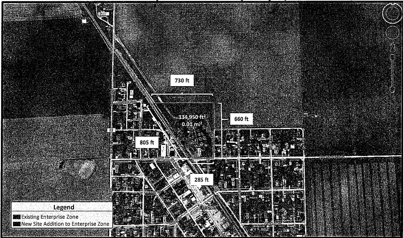
Site B Addition Satellite Map 2 – Grainland Coop Company Site in Emden, IL
